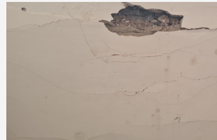
Ceiling cracks
