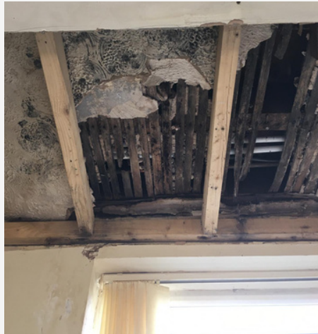
Severely damaged ceiling
