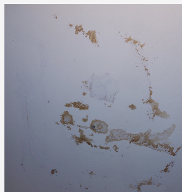
Leaking ceiling
